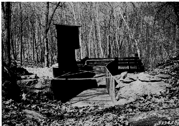
Figure 2.—Parshall flume with instrument shelter and silt collecting box, Watershed "B", Upper Mississippi Valley Soil Erosion Station, 1936.
