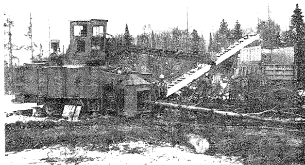
Figure 3.—USDA Forest Service, Missoula Technology and Development Center precommercial prototype wood chunker.
