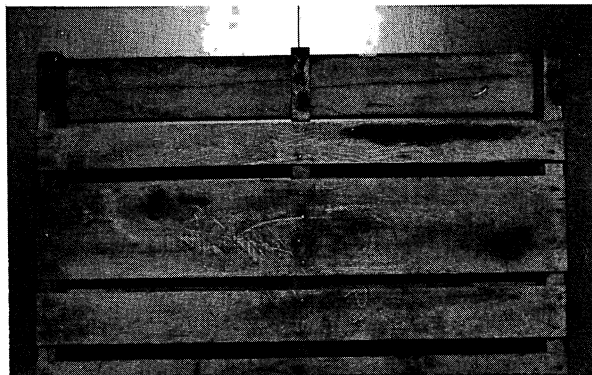
FIGURE 6.—Long, deep, continuous checking on upper surface of bottom edgeboard.
