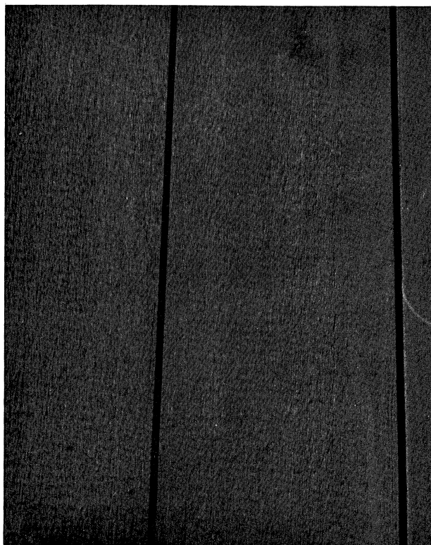
Figure 8.—Yellow-poplar tongue-and-groove siding, water repellent treatment on the south wall. The boards have shrunk exposing 3/16 inch of tongue, but the joint is tight.
