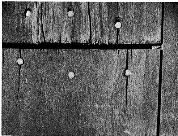
Figure 6.—This 1/4-inch butt joint gap in cottonwood tongue-and-groove siding resulted from excessive longitudinal shrinkage, particularly in the upper board. The indentation of the nail at upper right, and the splitting at nails is further evidence of longitudinal change.
