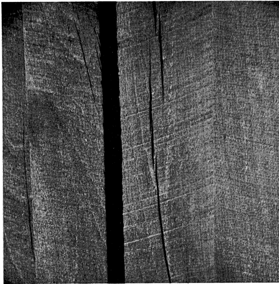
Figure 3.—Sycamore board-and-batten siding, untreated, south wall, with long mid-board splits.
