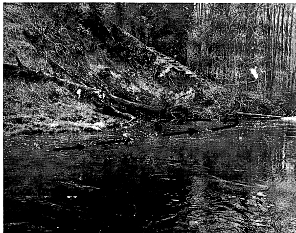
FIGURE 12. — Bank failure due to a rough transition between rip-rap and natural bank. The rough transition resulted in the eddy indicated by arrows.
