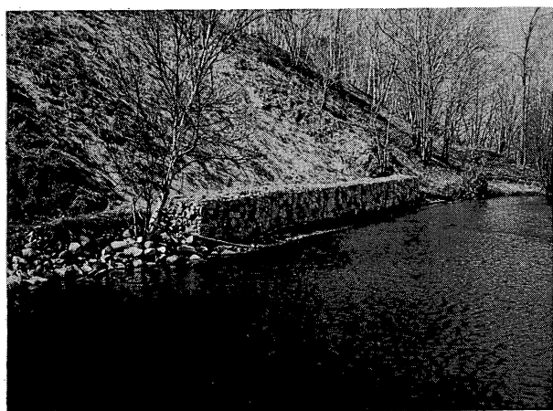
F-517759 FIGURE 10. — A gabion structure for controlling waterline erosion. The unnatural appearance may be undesirable in some situations.
