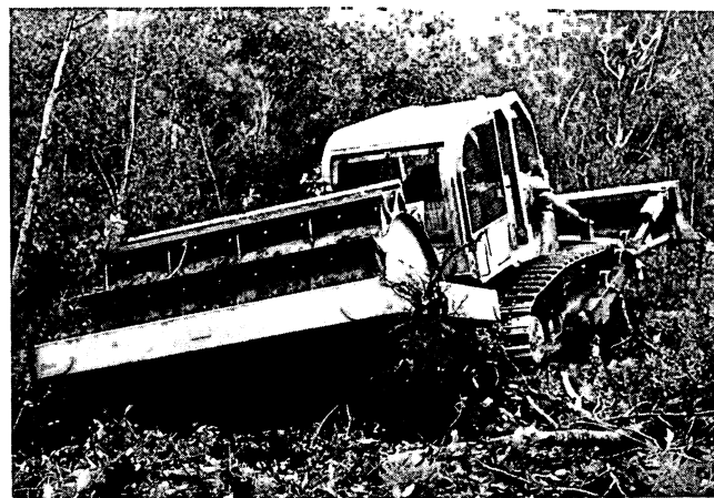
Figure 3.—Equipment used for roller chopping.
