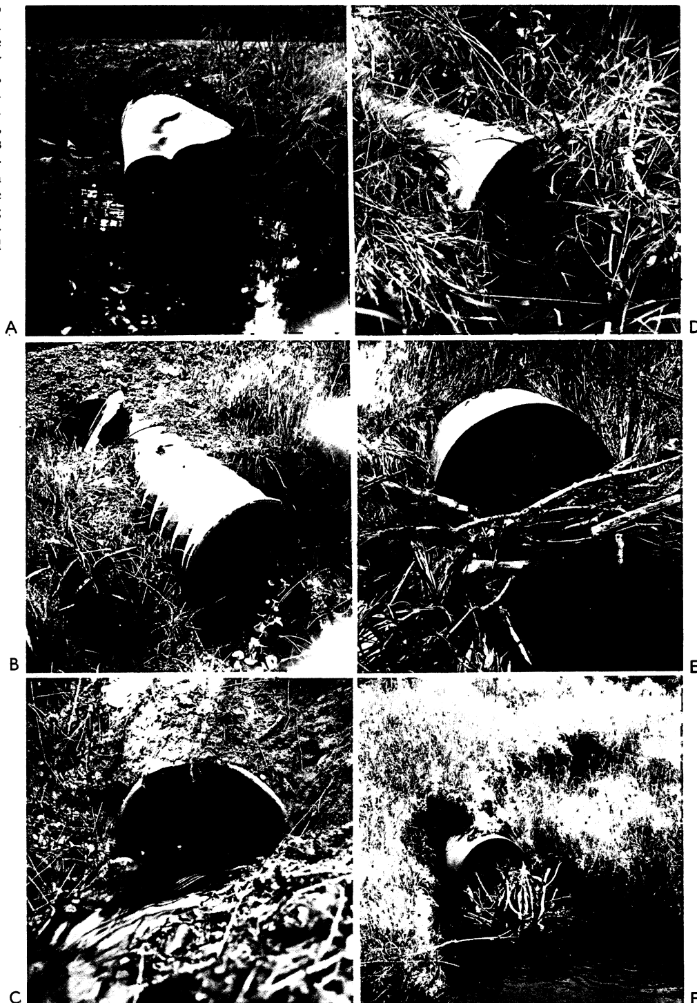
Figure 2.—A, culvert set too high, damaged by road grader; B, culvert intake capacity reduced probably by snowplow damage; C, culvert outlet half filled with gravel that sloughed off the road shoulder; D, grass, willow, and chunks of sod constrict culvert entrance; E, a culvert with about half its intake plugged with dry sticks; F, discharge end of a culvert partially plugged with sticks by beavers.
