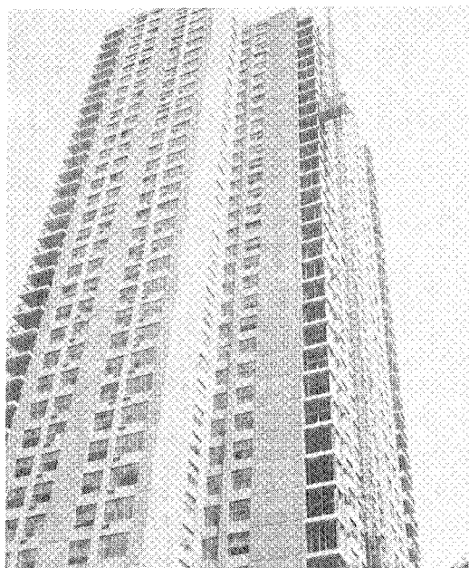
Figure 1.—The 39-floor high-rise tower studied in New York is provided with room air-conditioner openings in the avenue exposure side of the building.
