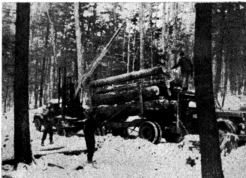
Figure 8.--Loader mounted on a separate truck.
