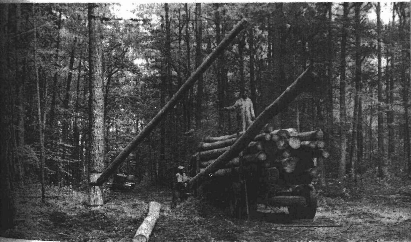
Figure 2.--A piling operation in Maryland. Above, peeled piling is skidded out of the woods by tractor.
