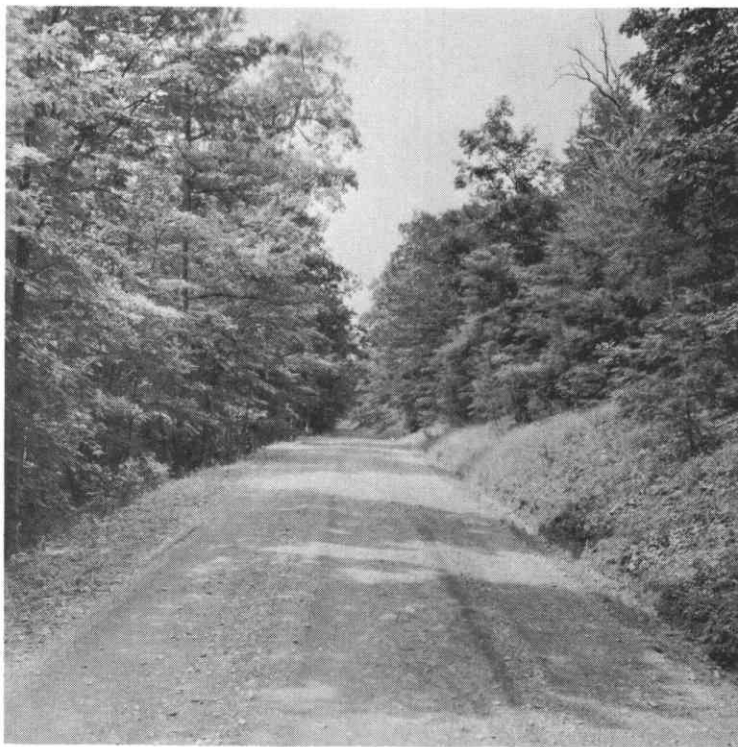
Figure 4.--A road on the George Washington National Forest 2 years after spraying in 1957. Shelf construction along a slope, with bank on one side and drop-off on the other, is typical of many forest roads. With selective oil-basal spraying, the bank remains stabilized under herbaceous cover. Compare this with Figure 1.
