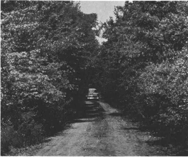
Figure 1.-- The need for roadside brush control. Without control of some sort, trees and brush encroach on forest roads, as shown by this town road in Maine. Cars are scratched, passing is made difficult, and visibility on curves is dangerously reduced.
