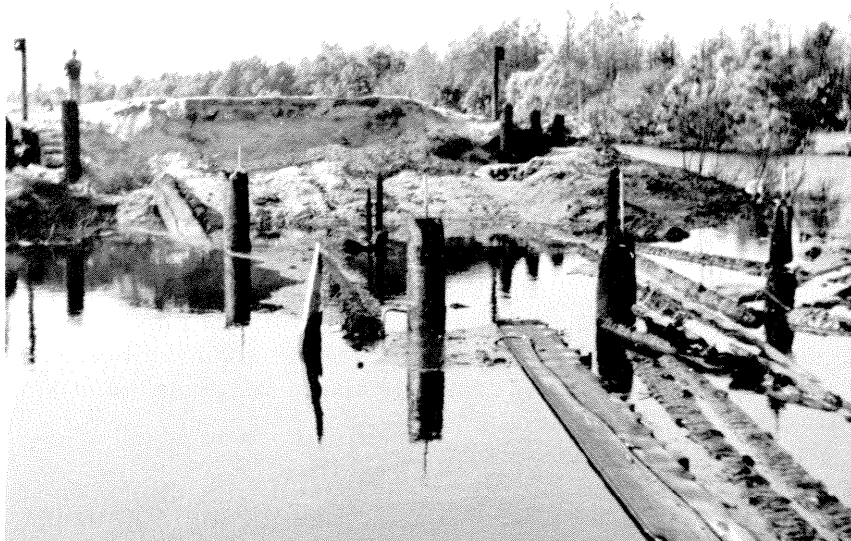
Figure 14. --Remains of a wooden bridge spanning a 30-ft.-wide (9-m.) canal along Navy Shell Road.
