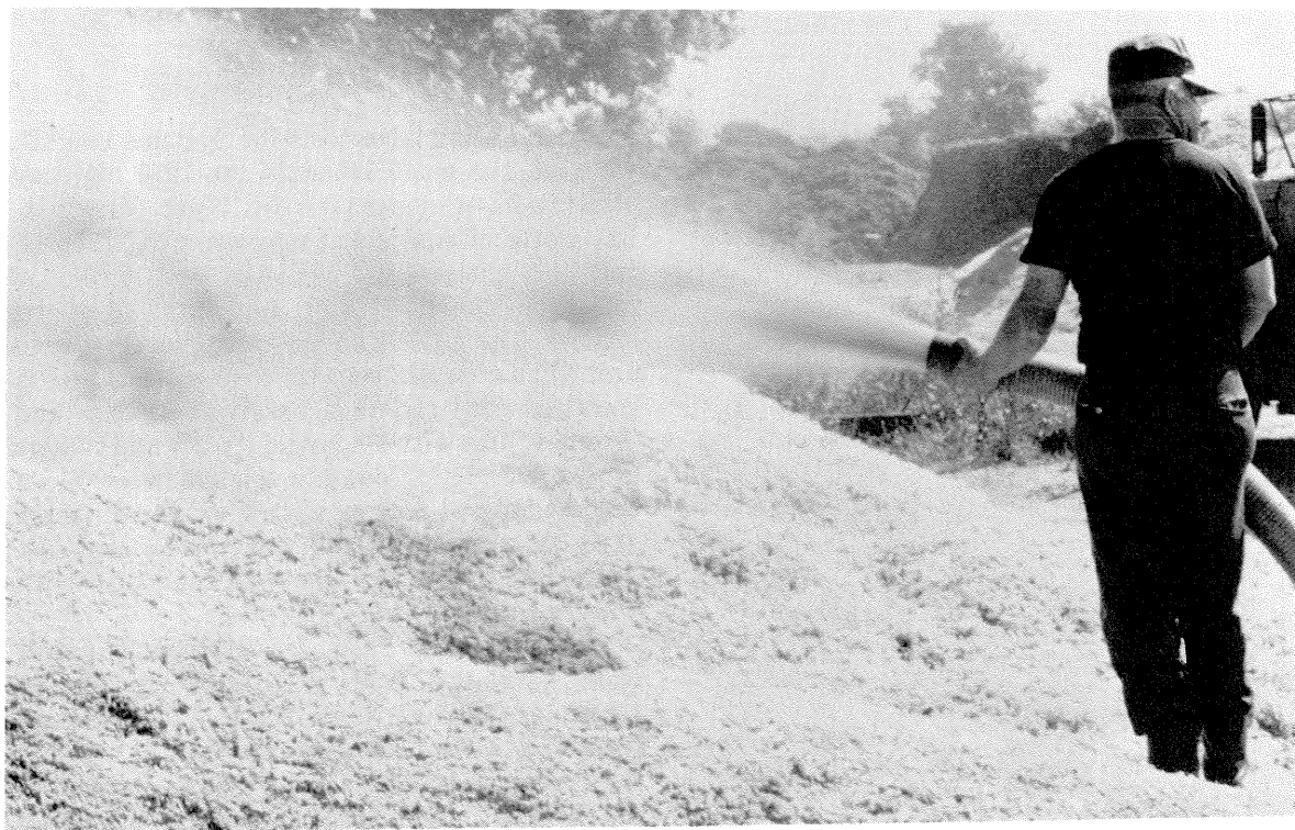
Figure 5.—MOBLOW handled dry, hardwood planer shavings exceptionally well; this material was blown as fast as it was fed into the system.
