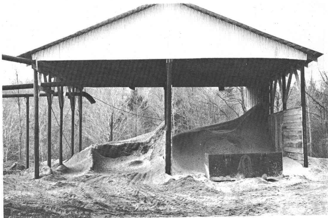
Figure 3.—Open pole-shed storage building for bark and sawdust. Bark is shredded and blown into compartment on left. Sawdust is blown into compartment on right. Material is loaded into open trailer van with 2½-cubic-yard rubber-tired bucket loader.
