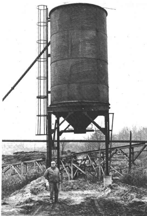
Figure 2.—A large steel tank used as a sawdust bin to load an open trailer van. Sawdust is trucked to Buffalo for the metallurgical industry.
