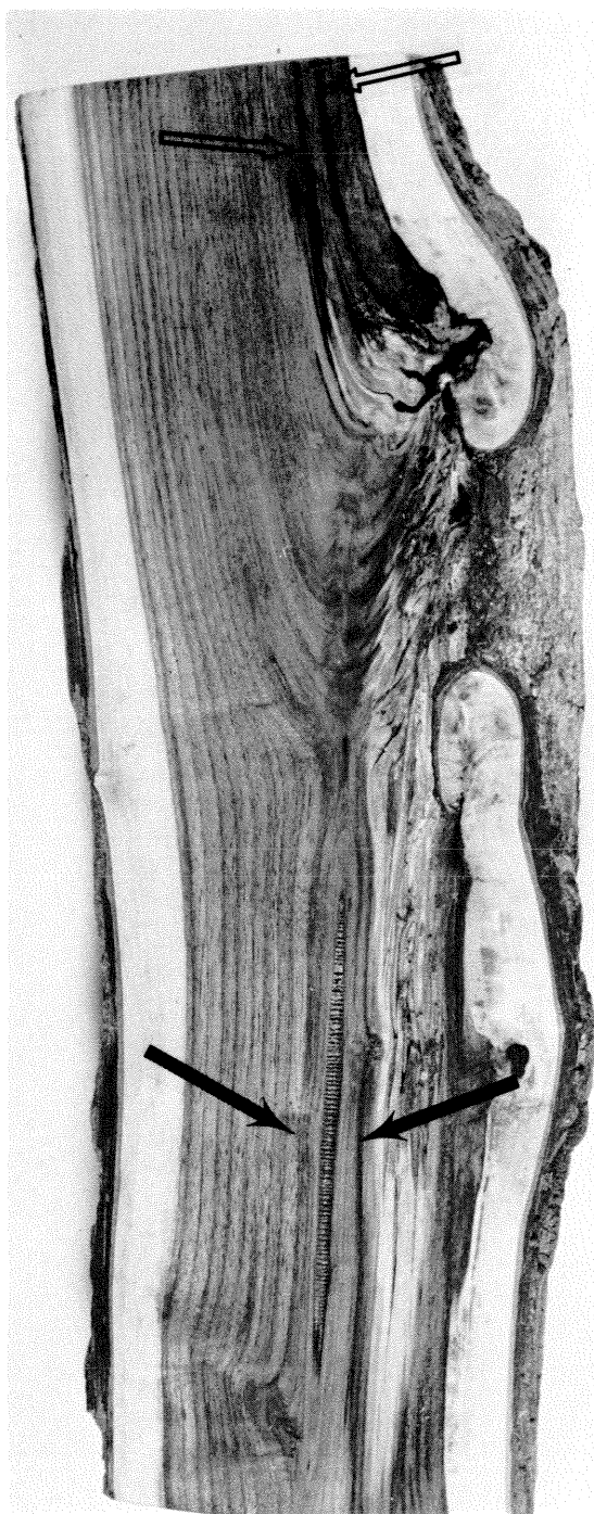
Figure 19.—Advanced decay associated with a large open 13-year-old pruning wound on a very slow-growing tree. Note that the outer portion of the stub is decayed, but the inner core of the stub and the tree are still sound. The large arrows show the inner compartment of sound wood. Yet, the heartrot concept would lead you to believe that the center of the tree would be decayed before the
