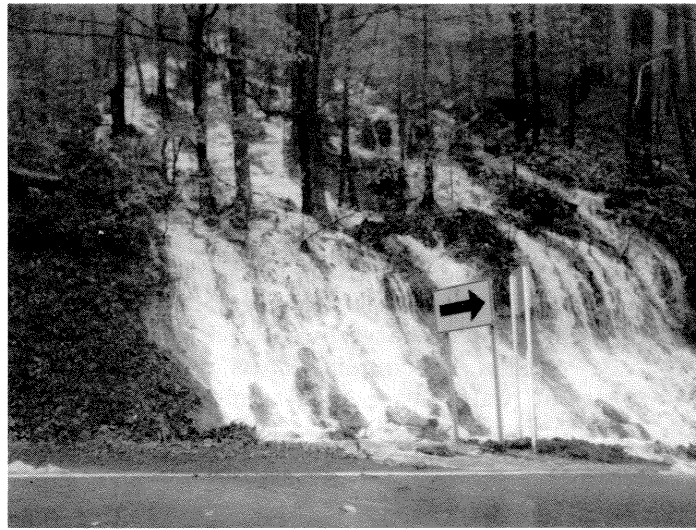
Figure 3.—Stormflow far exceeded the capacity of this ephemeral flow channel on Route 219. At this elevation (2,800 feet) tree foliage had only begun to emerge. Note small stones being washed along the road pavement.
