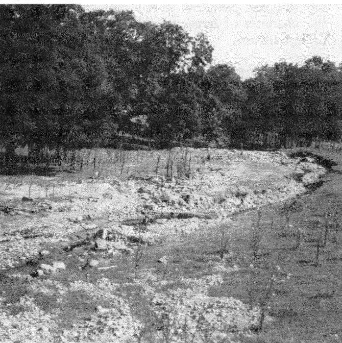
Figure 21. —The main channel of Johnson's Run, downstream from the outlets of gullies caused by road drainage.
