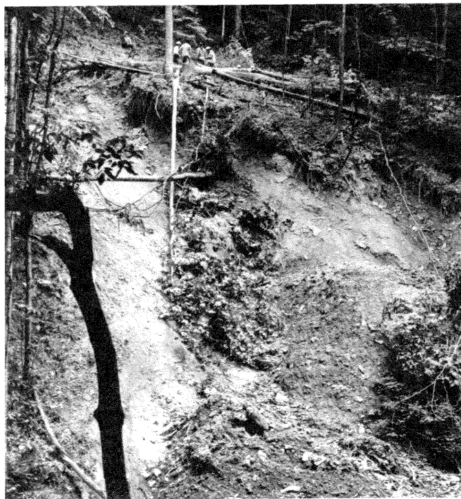
Figure 10.—Landslide on the Right Fork of Clover Run. The lightest colored surfaces are bedrock. For scale, note workmen at the top of the photograph.
