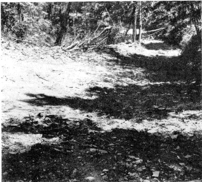
Figure 9.—View across a log landing, downslope along a logging road with an 8-percent grade. This road had not been regraded after the storm and presented no obstacle to safe driving.
