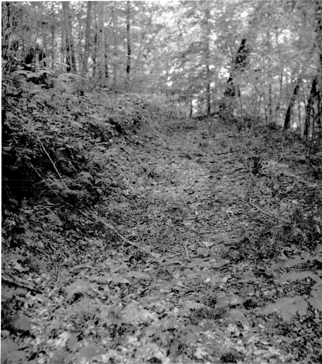
Figure 4.—This logging road, on an 8 percent grade, showed no sign of erosion after the storm of July 15 and 16.
