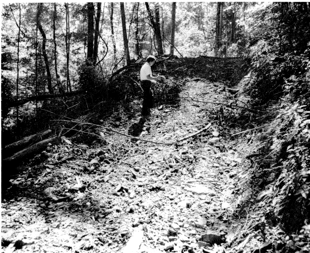
Figure 10.—The most severely eroded segment of the main haulroad, Bruffy property.
