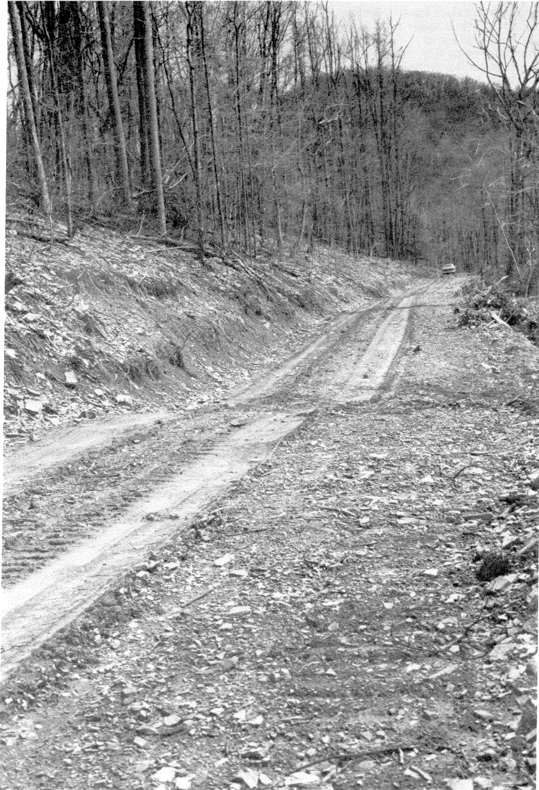
Figure 4.—Minimum-standard truck road with high content of natural coarse stone.
