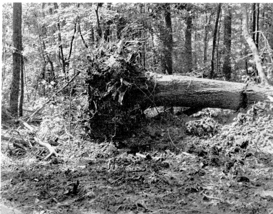
Figure 3.—Large tree removed on Road 5.
