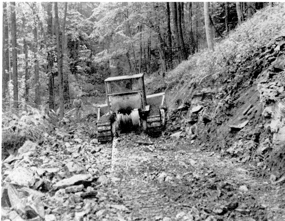
Figure 2.—Section on Road 5 where hard rock was encountered.
