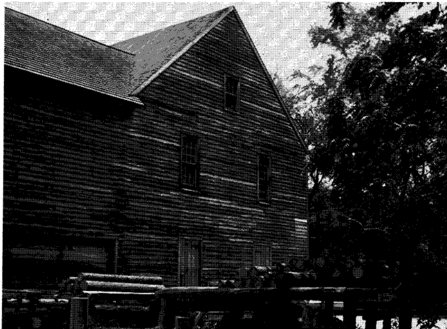
White-cedar logs ready for sawing.
