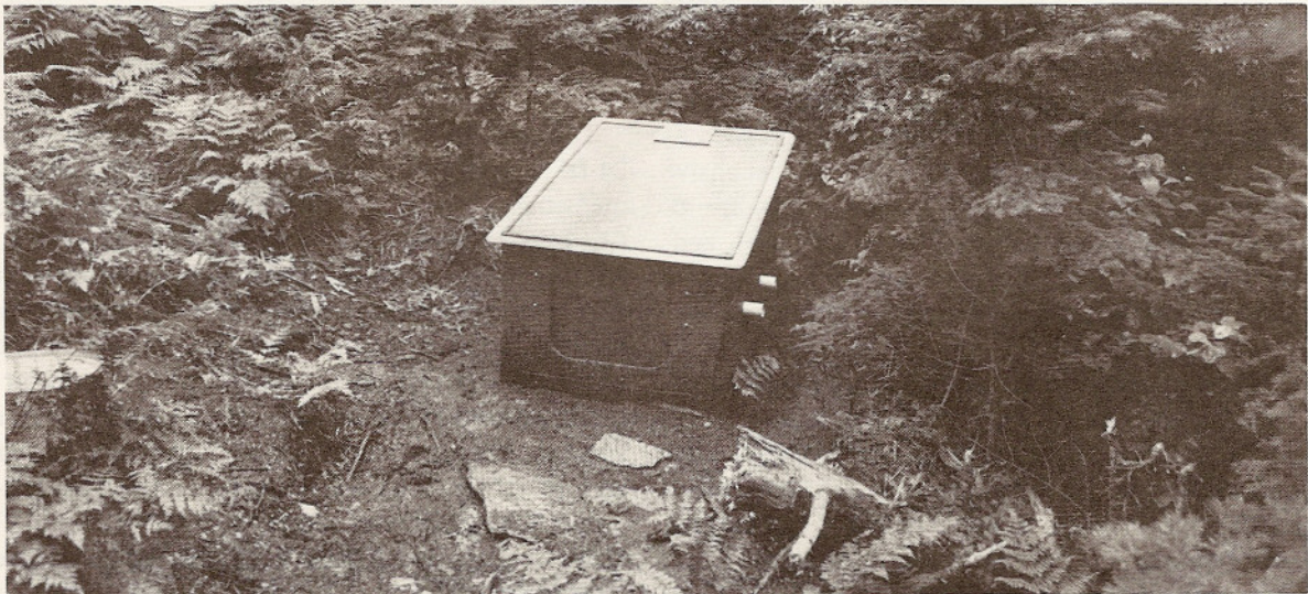
Figure 2.—The 24-ft 3 fiberglass Bin Composter.
