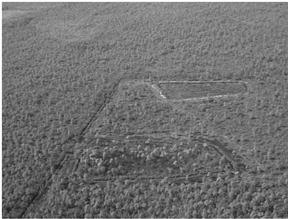
Figure 2.—Aerial view of two experimental pocosin burns in the Green Swamp. Only the surface fuels burned in the foreground. The burn unit in the back shows the peat burn unit one year after a burn.
