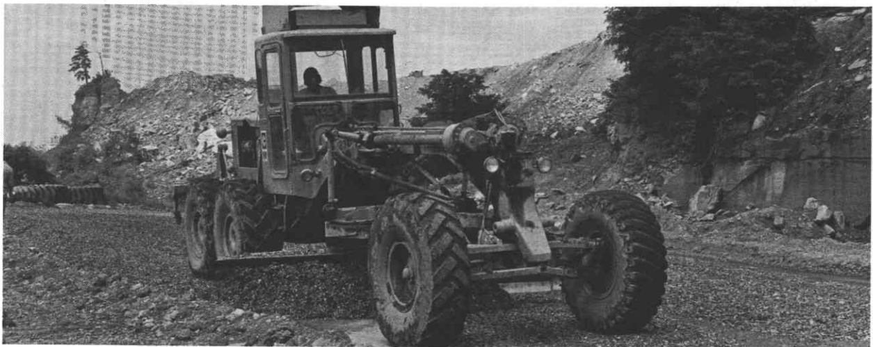
Figure 3.—Motor grader spreading wood chips into blanket covering road surface: 2:30 p.m. on first day.
