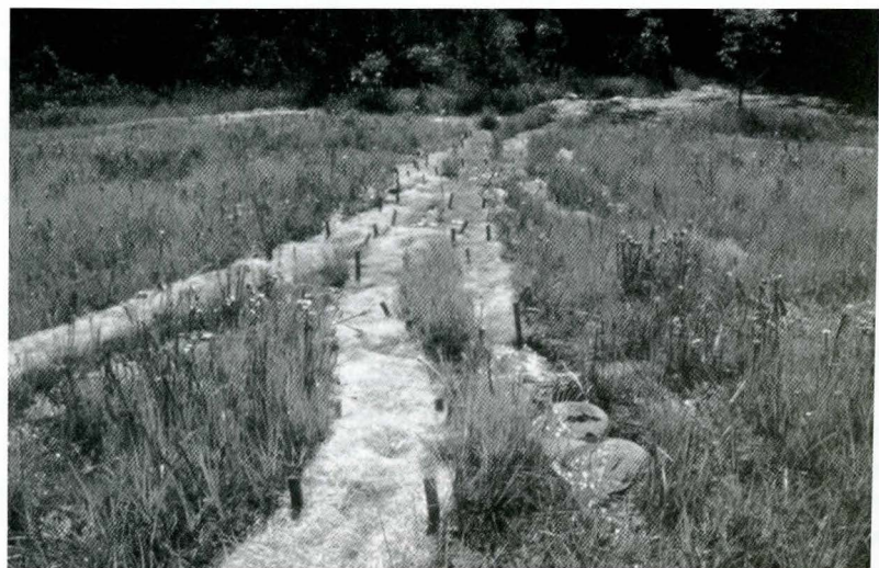
Figure 3. Phoenix bog on the Angelina National Forest, Texas, depicting restoration actions undertaken to restore the surface contours and stabilize the soil surface reducing the potential for erosion.
