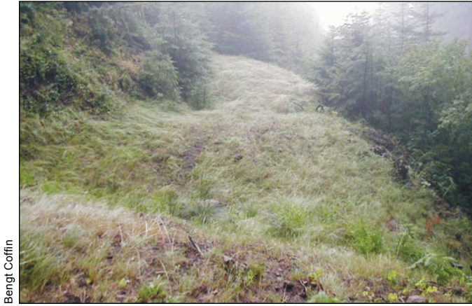
Figure 5—Decommissioned roads are stabilized and disconnected from natural surface hydrological features.
