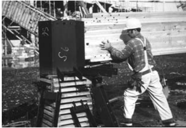
FIGURE 10.3 Large composite beam made from laminated lumber.
