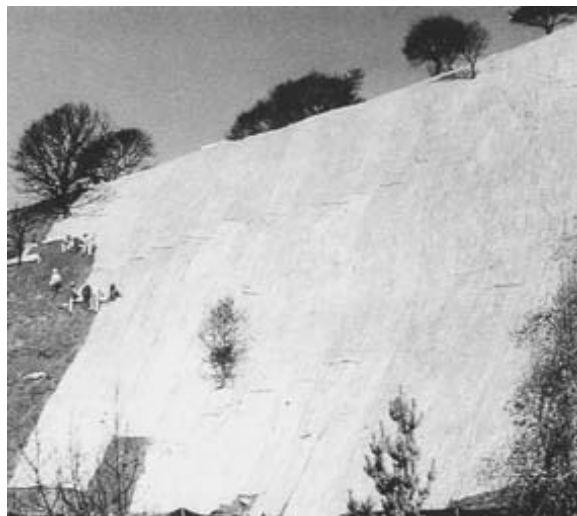
FIGURE 12.8 Application of fiber-based geotextiles.
