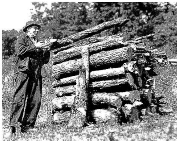
FIGURE 21 — These pictures show some of the work that went into making charcoal in years past. Upper is an area cleared for charcoal wood. In the center a worker is piling the wood on the cutting site. Lower, the wood has been hauled and piled at the burning site, and the workers are now covering the wood with dirt and leaves before lighting the fire.
