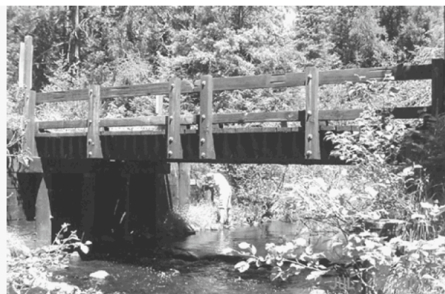
b) Side View of Bridge Deck
