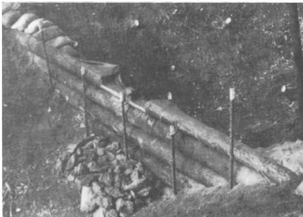
Downstream face of a typical dam. Large rocks placed below the spillway prevent formation of a plunge pool which could undermine the dam.
