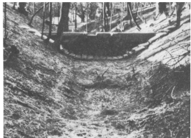
Upstream face of a completed dam. Natural channel has been widened to increase reservoir capacity. Sandbags secure the reinforced silt cloth to the bottom of the reservoir.
