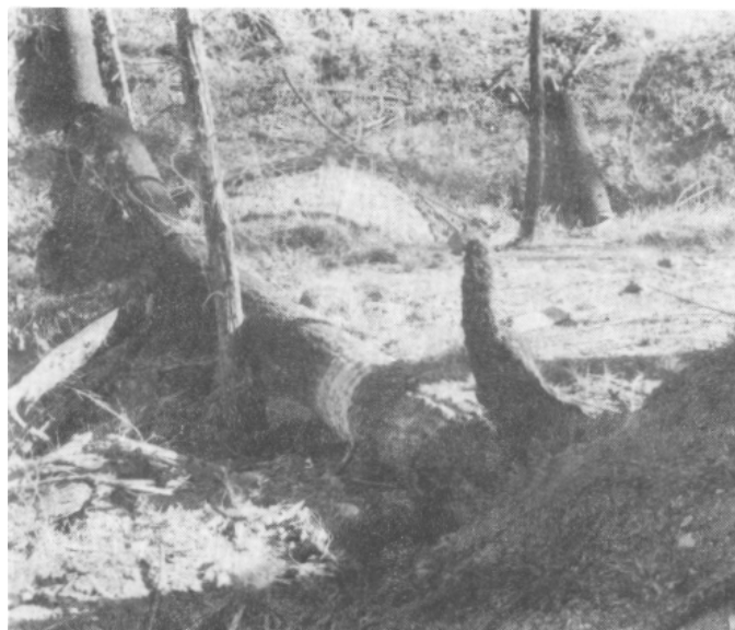
Figure 5--Typical log and straw bale retention structure in one of the smaller drainages. Note accumulation of sediment behind structure.
