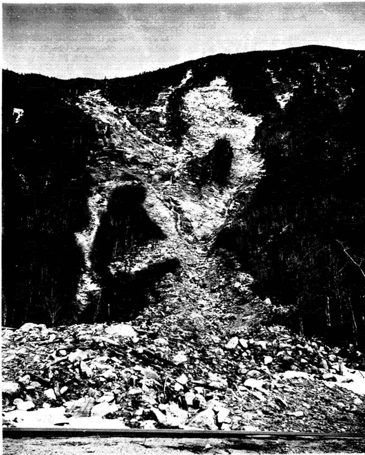
Figure 2.—A recent landslide in Franconia Notch. Deciduous trees colonize these new slide areas and conifers follow much later. The sites of older landslides are marked by deciduous trees in the photograph.
