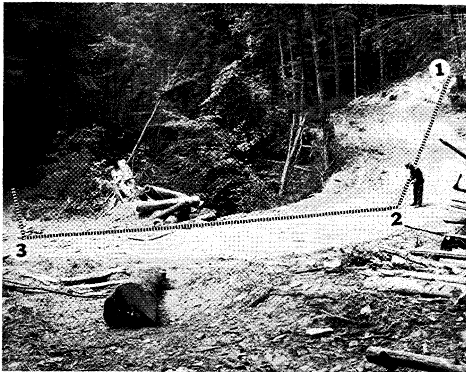
Figure 2.—Technique of measuring alignment segment lengths. Line of sight follows dotted line.
