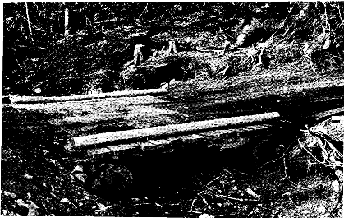
Figure 17.—A logging-road bridge, suitable for crossing small streams, made from low-grade hardwood lumber and nearby trees. This bridge easily supported a 15-ton bulldozer and will carry loaded logging trucks for several years.
