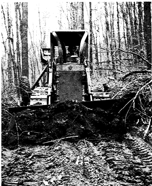
Figure 19. — Waterbars being installed on a logging road to be closed to all vehicle traffic.
