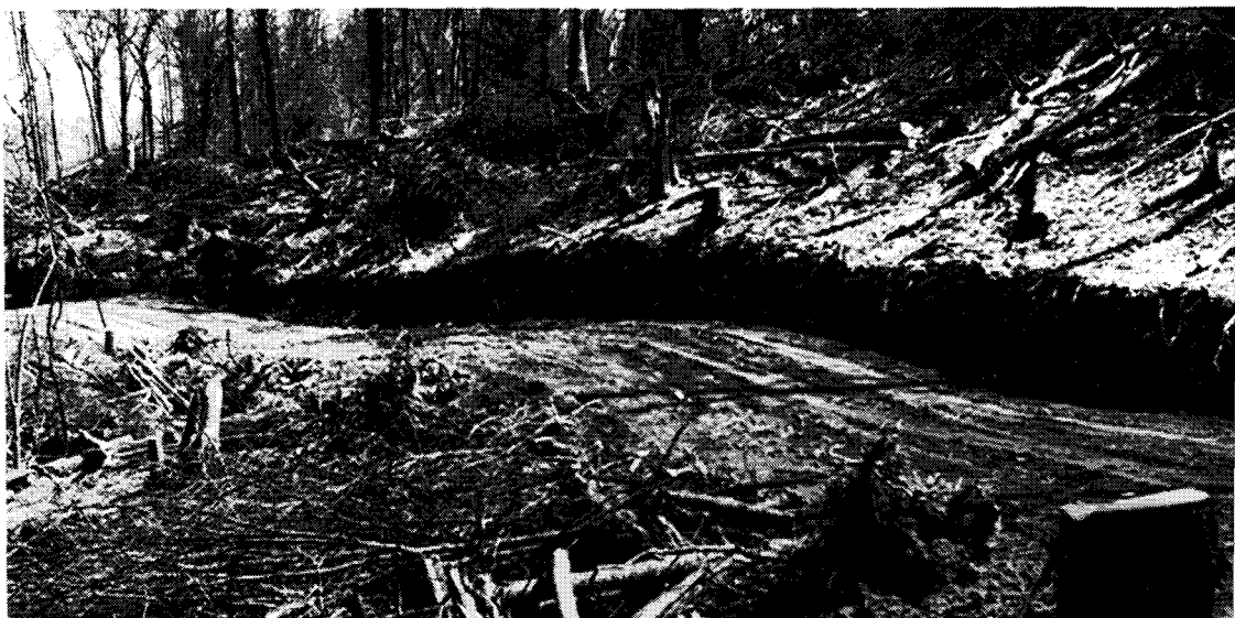
Figure 15.—Properly constructed broad-based drainage dips are cheaper to maintain and more permanent than wooden culverts.
