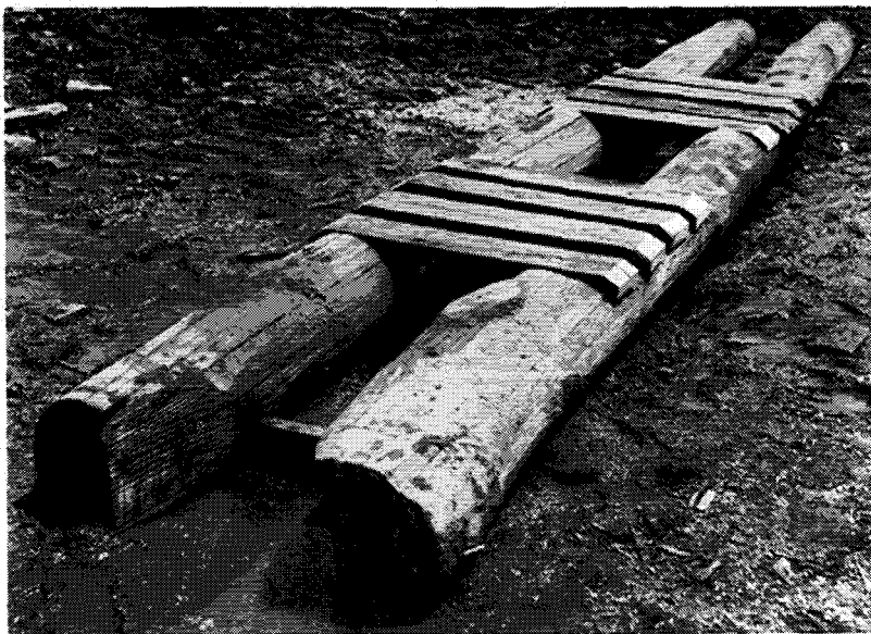
Figure 12.—This type of open-top culvert does not become plugged with debris as readily as ordinary open-top culverts, and the cost for materials is less. Note the spreaders on the bottom of the logs to prevent them from becoming squeezed together, and the 2-inch spaces between the boards to prevent water from running down wheel tracks and across the culvert. This same principle can be used to construct closed-top culverts.
