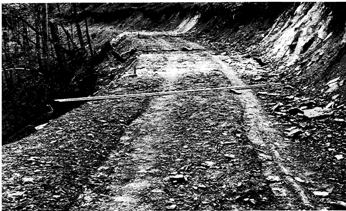
Figure 8.—A properly located and properly constructed logging truck road. The road is on a hillside and is well above a stream. The long climbing grade is broken by culverts, and the roadbed contains a high proportion of natural stone.
