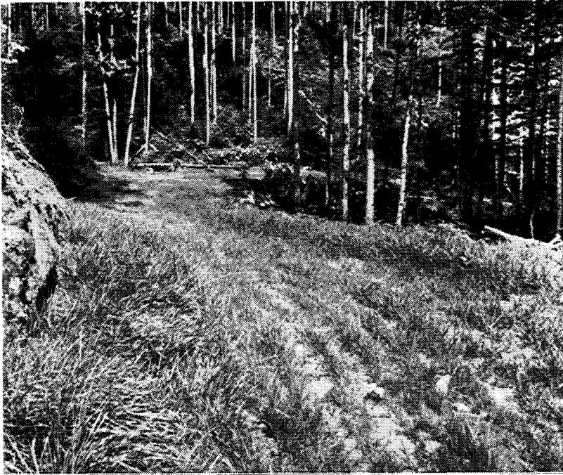
Figure 21.—Seeded logging roads help control erosion.
