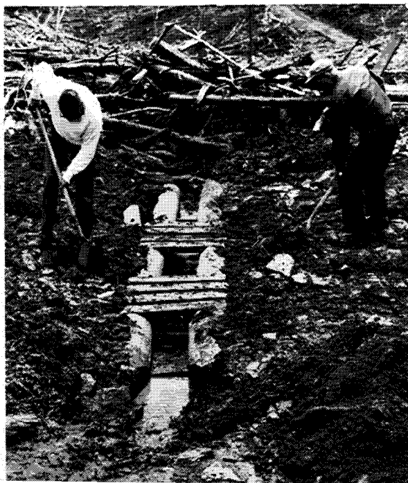
Figure 13.—Proper installation of culvert shown in figure 12.
