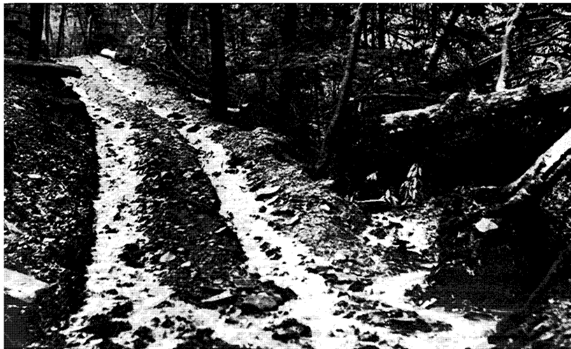
Figure 3.—Excessive erosion and costly damage caused by poor logging-road location and lack of adequate drainage.
