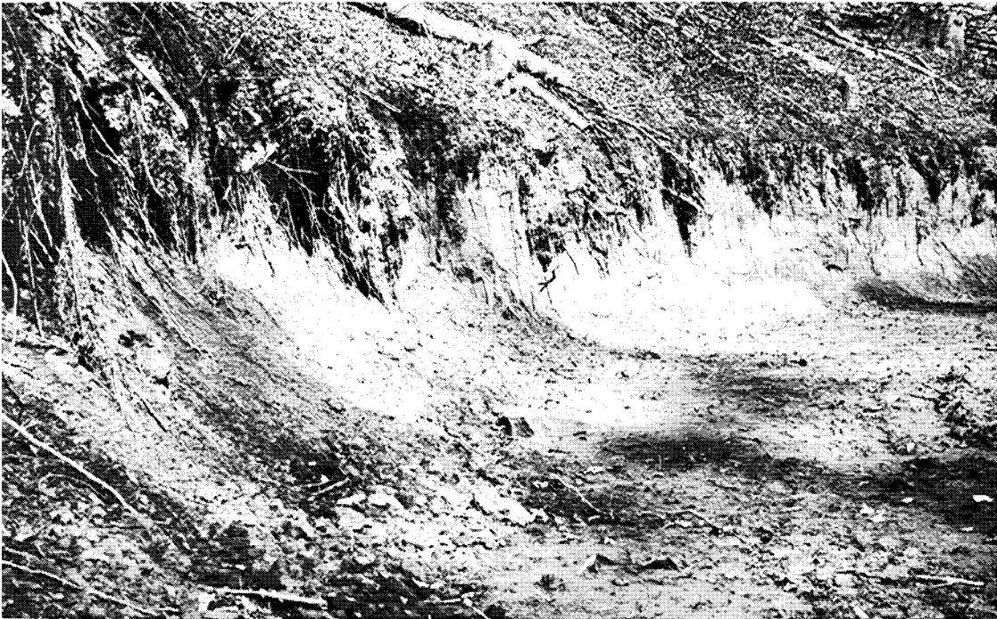
Figure 2.—Roadbuilding removes the litter that protects soil against erosion.
