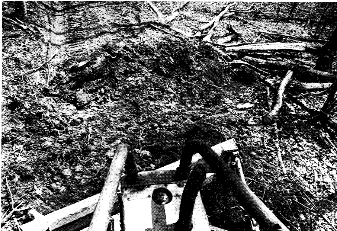
Figure 20.—A properly constructed waterbar.
