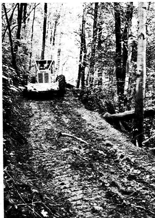
Figure 7.—Well-located and well-constructed roads with gentle grades are required for the efficient operation of modern logging equipment in the rugged Appalachian Mountains. Because these wide roads expose more soil than the narrower roads formerly used, careful erosion control is important.
