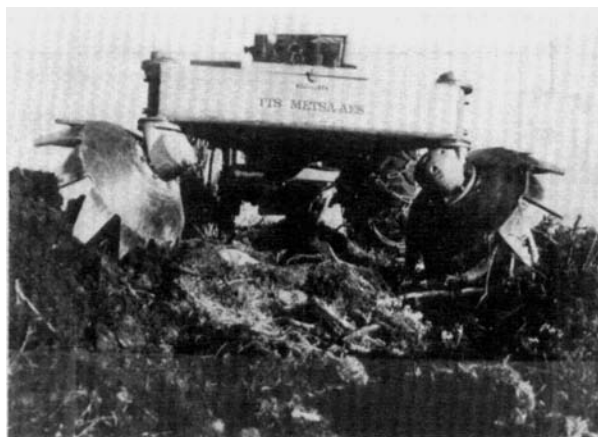
Figure 3.—TTS disc trencher
