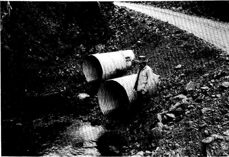
Figure 17.--These culverts were improperly installed above the streambed and will not allow upstream passage of resident coho and trout. Kuiu Island, Alaska, 1975. (Photo, courtesy of Alaska Department of Fish and Game.)
