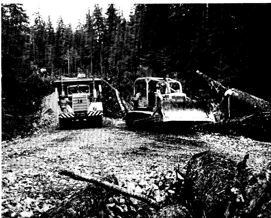
Figure 16.--A typical rock-overlay logging road under construction on Prince of Wales Island, Alaska.
