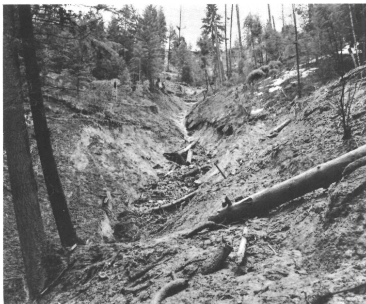
Figure 3-c. Debris torrent developed in an intermittent stream channel along the South Fork of the Salmon River in Idaho. Initial failure occurred in road fill near the ridgetop.
