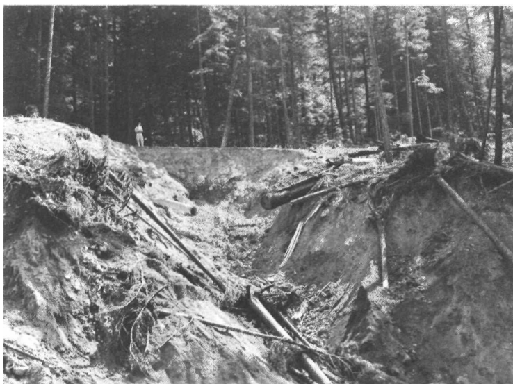
Figure 6c. Failure due to inadequate road drainage in the Cascade Range of Oregon.
