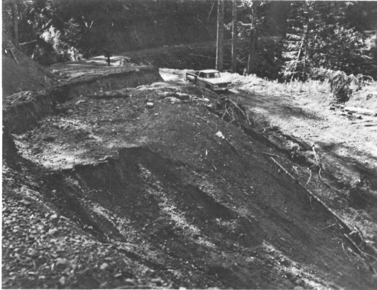
Figure 6. Examples of mass soil movements resulting from failure along a road right-of-way, a) Road fill failure in the Cascade Range of Oregon. Failure resulted from plugged side drainages and resultant saturation of the road prism.
