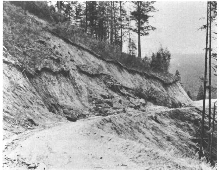
Figure 6b. Backslope failure along a logging road in the Salmon River Mountains of Idaho. Failure resulted from undercutting of the slope toe.
