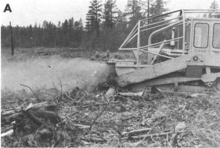
Figure 3.-- Tree Eater operation on Deschutes National Forest: A, Treating logging residue prior to planting seedlings: B, appearance of residue after treatment.
