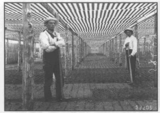
Figure 1. Horizontal overhead snow-fencing, "Pettis frames".
