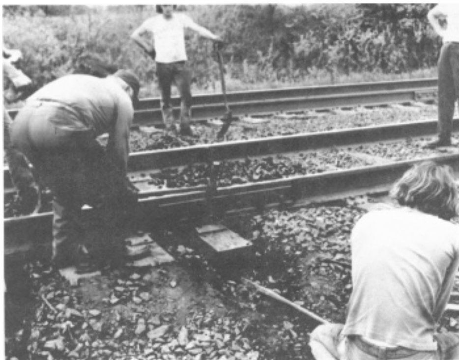
Figure 1.—Press-Lam crosstie being placed in track
