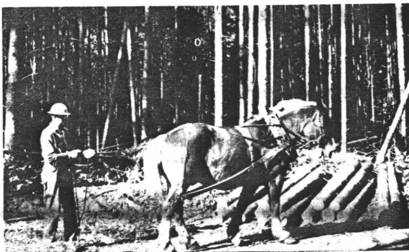
Figure 1.--Logs are skidded by horse and bunched along road preparatory to loading.
