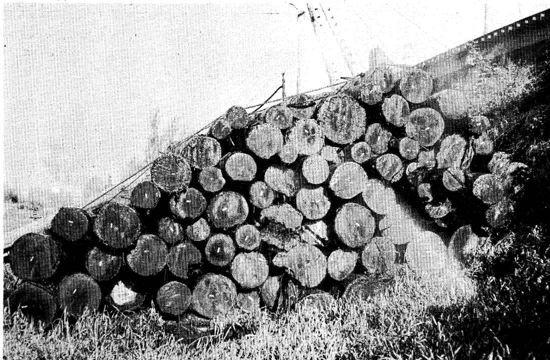
Figure 1.--Sprinkled hemlock log deck near completion of the test. The manner of decking is typical of the way logs are commonly stored for a year or more in the Pacific Northwest, but the pile is considerably smaller than the average found in industry. Note sprinkler atop deck.
