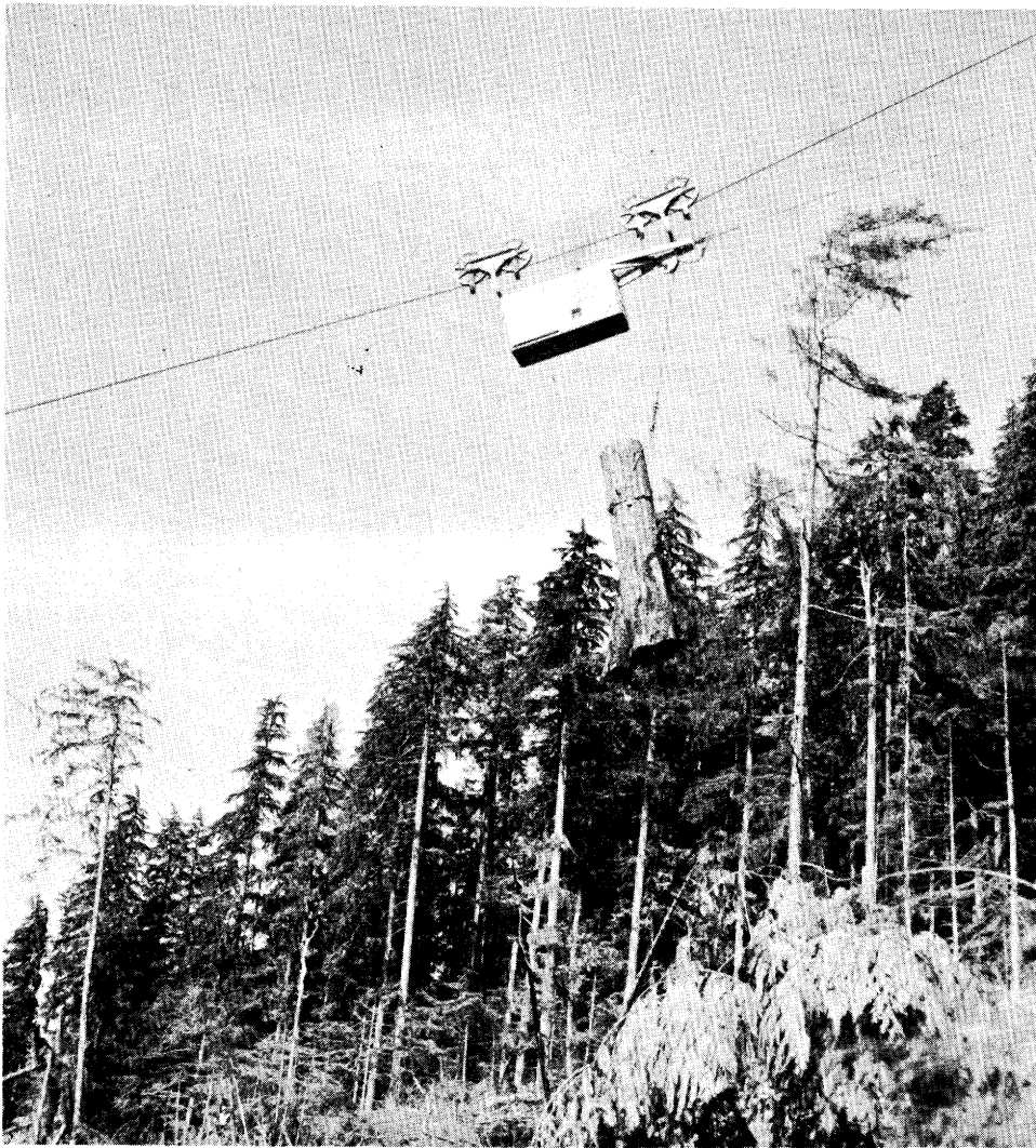
Figure 1.--A radio-controlled carriage in operation on the Mount Baker National Forest. Logs are yarded to the skyline by an engine in the carriage; then the carriage, controlled by a winch at the top of the hill, moves downhill by gravity. The skyline span is 5,000 feet, and lateral yarding to the skyline is effective up to 200 feet.
