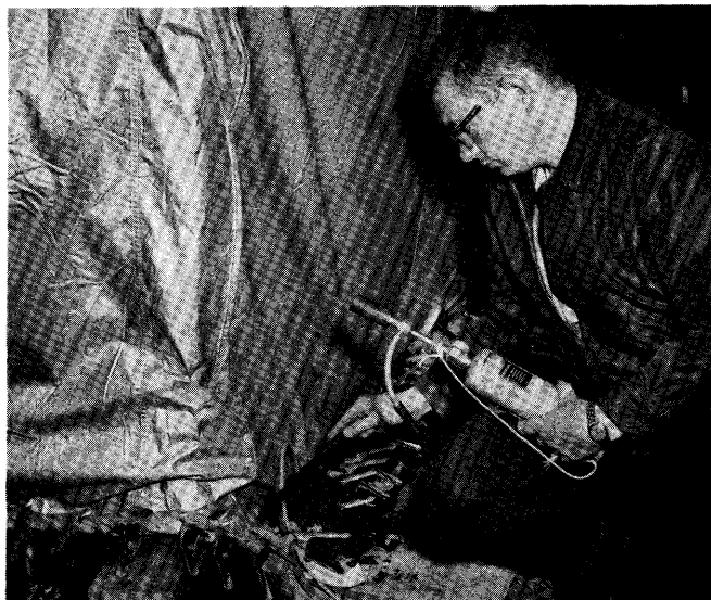
Figure 3. - Searching for gas leaks with halide detector.
