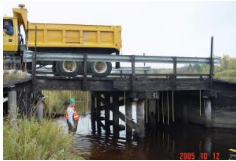
Fig. 1 Static live-load testing.
