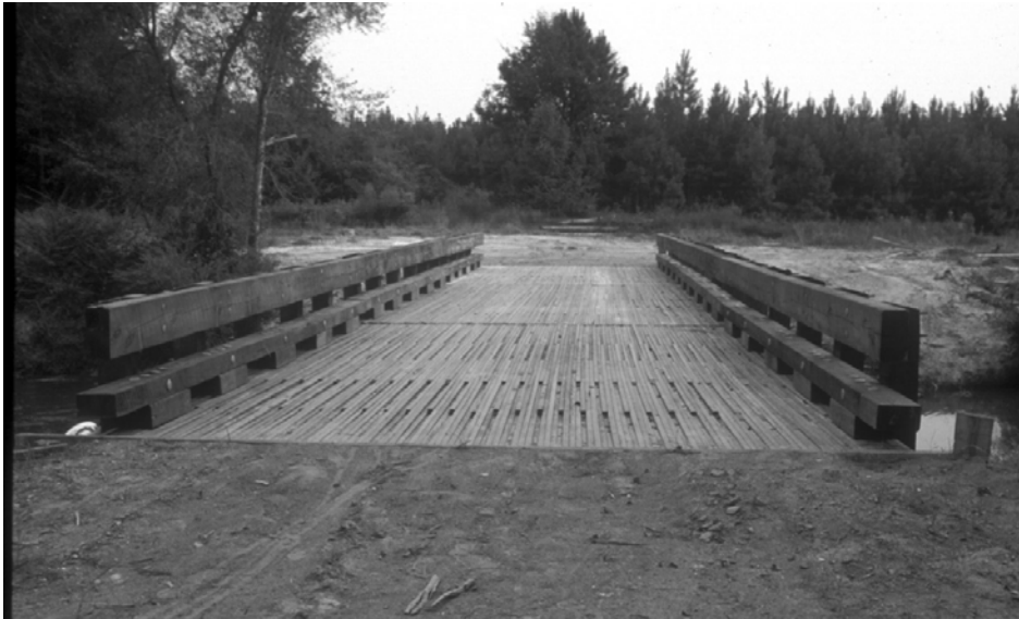
Figure 1: Spirit creek bridge after installation in 1991.
