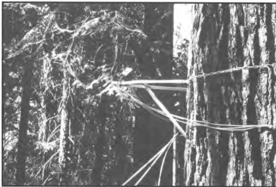
Figure 6--(b) An "A" frame bracket on the tree holds the octopus and extension cable junction boxes away from the tree surface.
