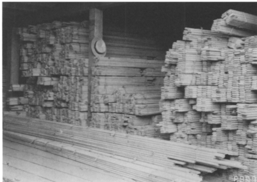
Figure 2-- Tanoak strip flooring manufactured by Union Lumber Co., around 1910, is ready for installation. (USDA Forest Service photo)
