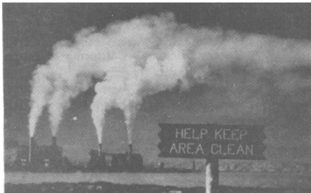
Figure 5--Stack emissions from Four Corners power plant.
