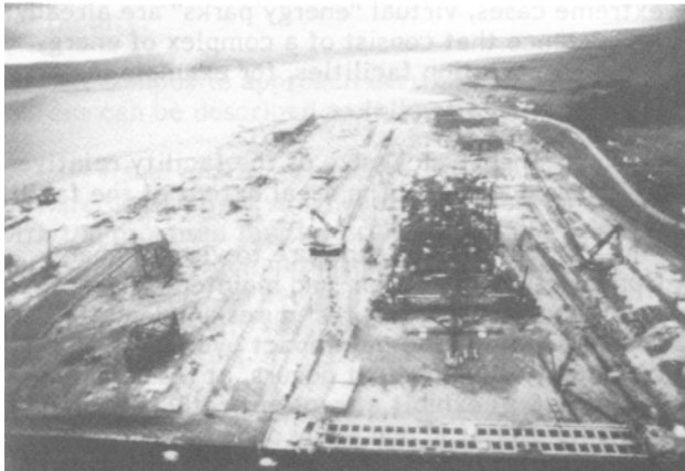
Figure 2--Platform fabrication yard.
