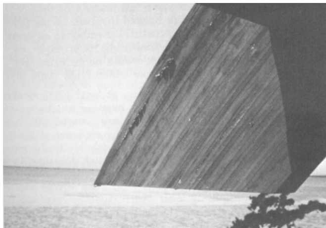
Figure 1--Mushrooms on exterior glulam (courtesy of W.A. Dost).
