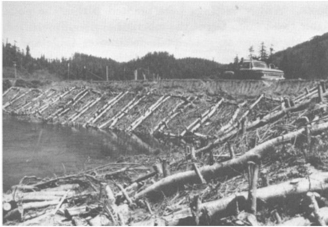
Figure 2 — Bank stabilization along Prairie Creek. Willow logs and hog wire were staked to what was a bare, eroding streambank. January 1984.
